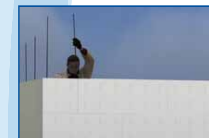
INSERTING THE REINFORCEMENT RODS
