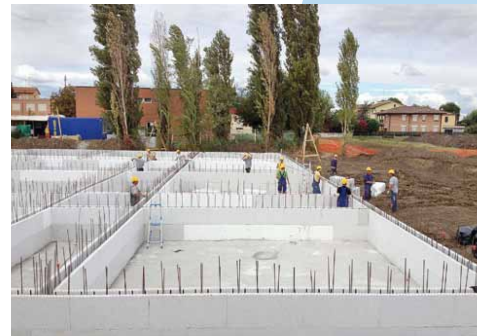
INSERTING THE REINFORCEMENT RODS
