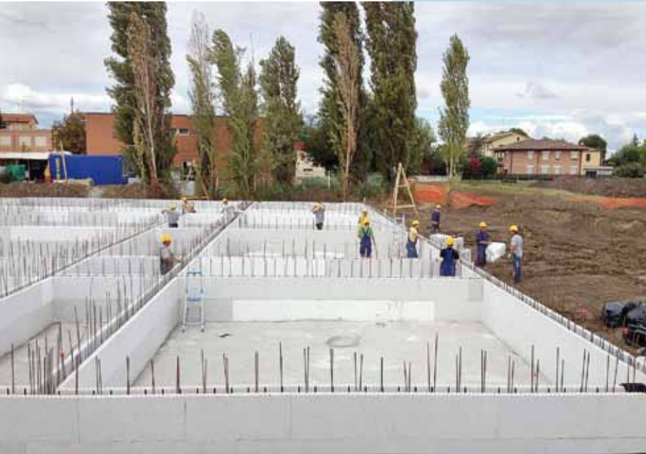
INSERTING THE REINFORCEMENT RODS
