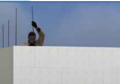
INSERTING THE REINFORCEMENT RODS
